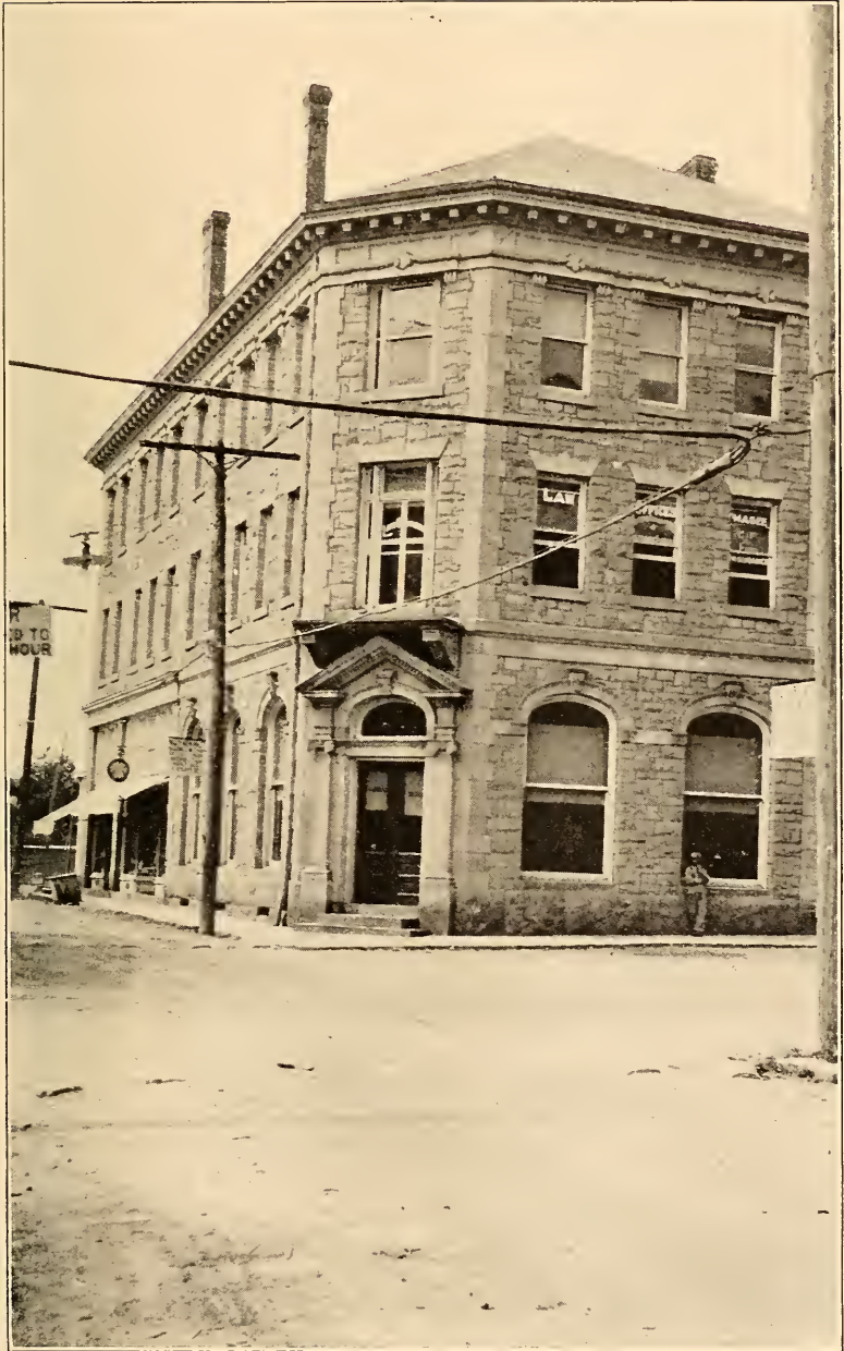
PLATE XV.—View showing Fayette County National Bank building at Fayetteville, constructed with stone obtained at local quarries in Upper Nuttall Sandstone ledge.
